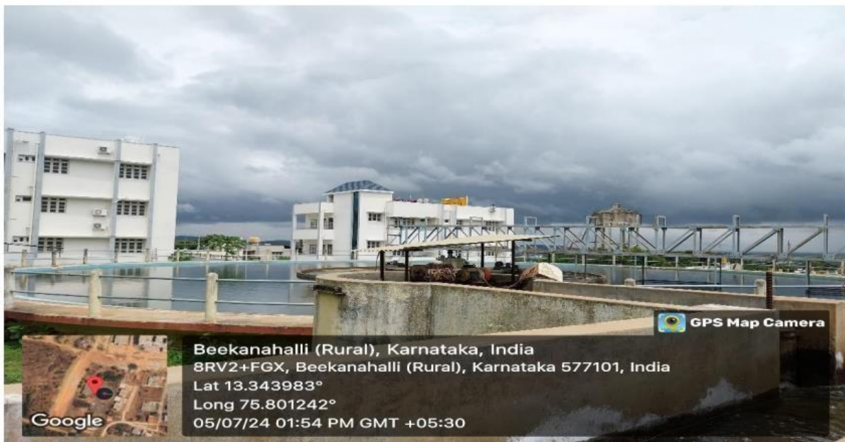
Fig 1.3: Water storage tank
