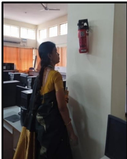
Safety measures at AIT, Chikkamagaluru, Karnataka
