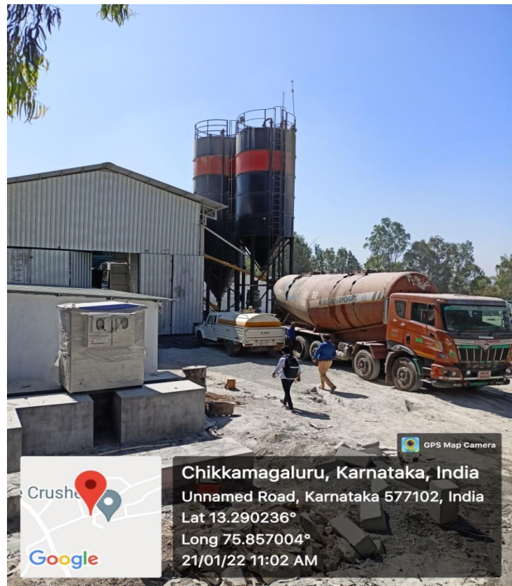
Photo of Cement dumping to Silos from Truck
