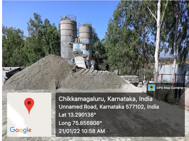
Photo of Materials and Silos
